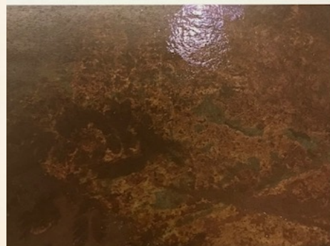
Floor during clean out
