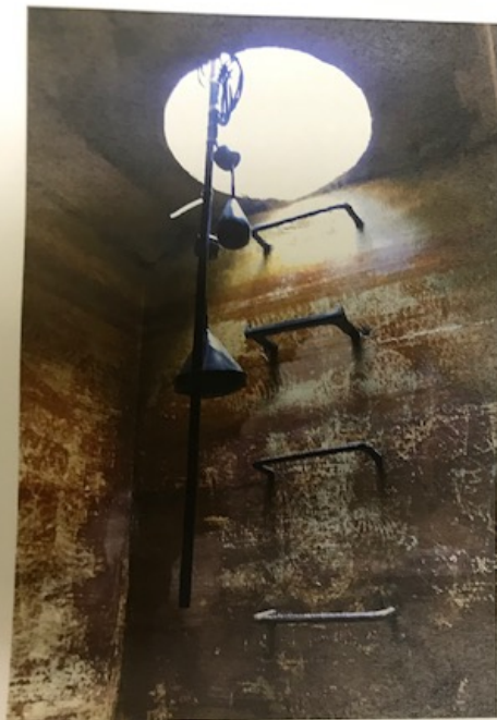
Ladder and controls
