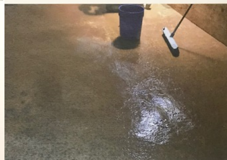
Floor after clean out
