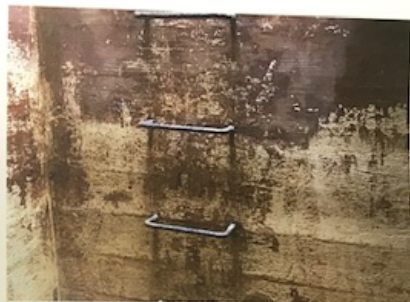
Access ladder and walls
